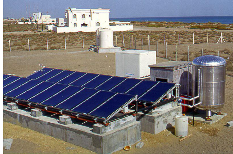
PV- and wind-powered reverse osmosis
